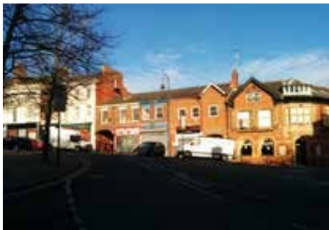
Left: Existing buildings to the eastern edge of Market Place
